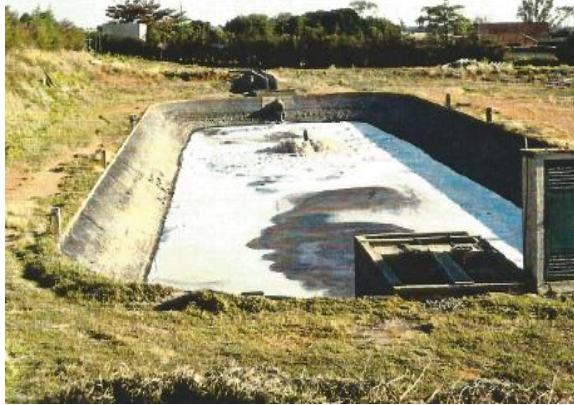
Fig. 15. Aeration pond receiving the effluents generated during the leather production in tanneries in the Franca region. According to [10].
