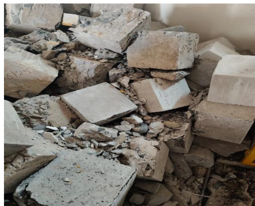
Fig-3 Concrete demolished waste
