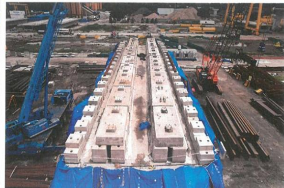
Placing of Concrete blocks (Type-1&3) On the FSLM Girder for completion of 75% test load
