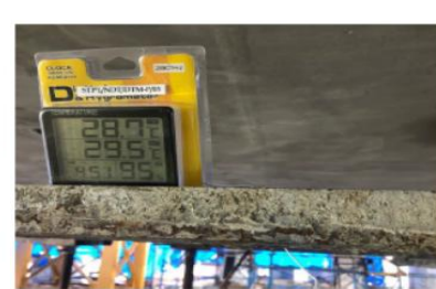
View of Digital Thermometer placed closed to the FSLM girder for measurement of ambient temperature
