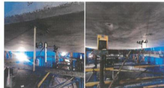
View of Independent HD Towers at Mid span (L/2) for placing of LVDT's and Dial Gauges
