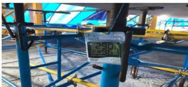
View of Digital Thermometer with External sensor firmly fixed to the soffit of FSLM Girder of Deflection measurement region.
