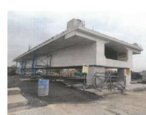
View of FSLM Box Girder with whitewash supported on RCC Pedestals
