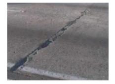
2. Faulting: A diffrence in elevation across a joint or crack usually associated with undoweled slab. It is noticeable when the average faulting in the pavement section reaches 2.5 mm, when it reaches 4mm diamond grinding or other rehabilitation measures should be considered.
