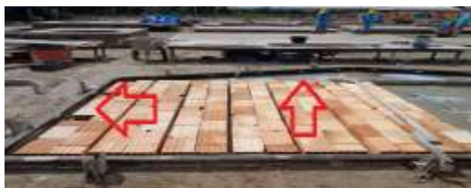
Figure 3: Details of the concreting regions for fixing the hooks.
