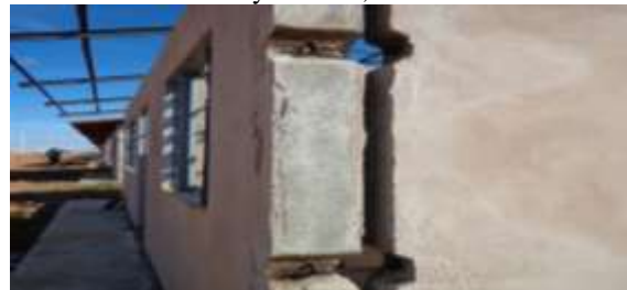
Figure 9: Locking the structure.
