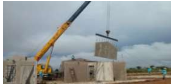
Figure 8: Mounting the masonry on the radier.
