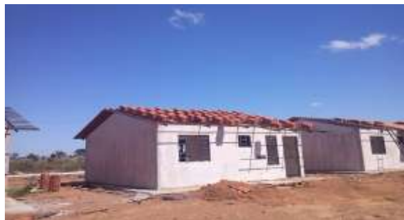
Figure 10: Roof over metallic structure.
