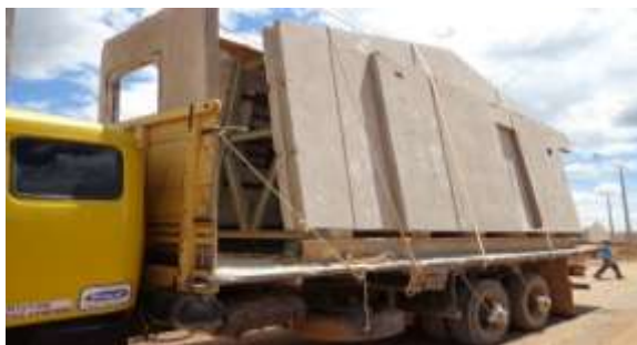
Figure 7: Transport from the precast wall to the radier.
