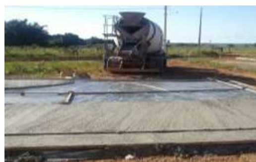
Figure 1: Concreting of the radier.
