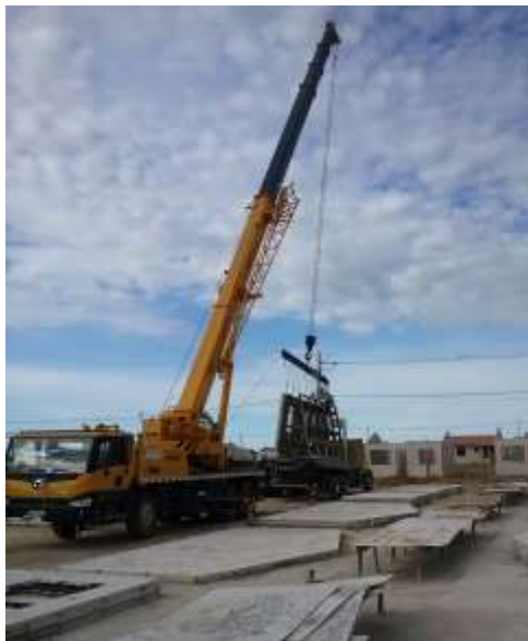
Figure 6: Lifting the precast wall.
