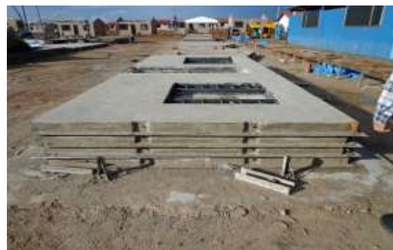
Figure 5: Finished wall for transportation.
