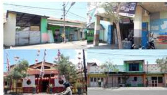
Figure 5. Types of Building Functions in the Ampenan Old Town
