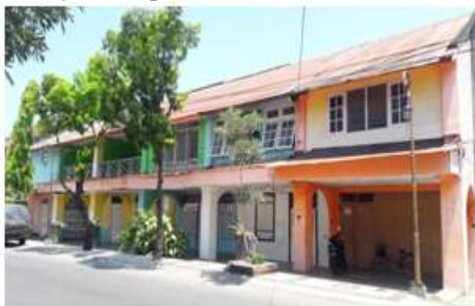
Figure 3. Buildings in the Ampenan Old City
