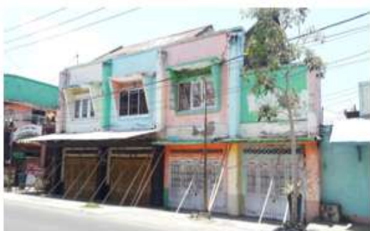
Figure 4. Buildings Damaged by Earthquakes
