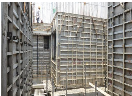
FIG 4.1: - Construction using mivan technology
