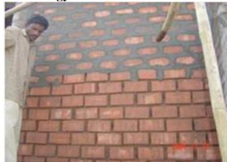
The Wall: Ordinary Mud (80% Murrum & 20% Bc Soil Or Clayey Soil) Is Used To Make 230 Mm Thick Walls Using Tile Faced Mud Blocks Of 100 Mm Thick And Filling The Masonry Joints With Cement Pointing. The Mud Block Wall Is Rain Proof And Rodent Proof. This Is To Be Noted That There Is No Need To Press Or Ram Or Concrete Or Add Any Other Binding Material In These Blocks.
