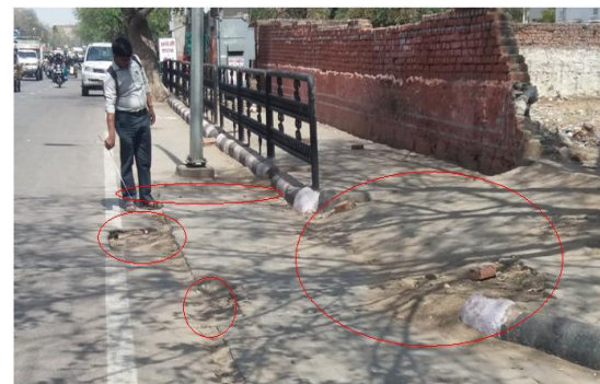
Figure: 2 Discontinue kerb at footpath
