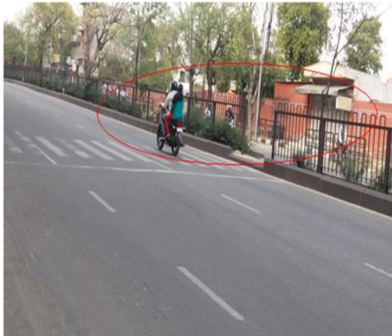
Figure: 4 Irregular opening of Guard Rail at Kalyan Nagar
