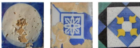
Figure 2: Different levels of degradation of tiles of facades with falling of glazed in Lisbon.
