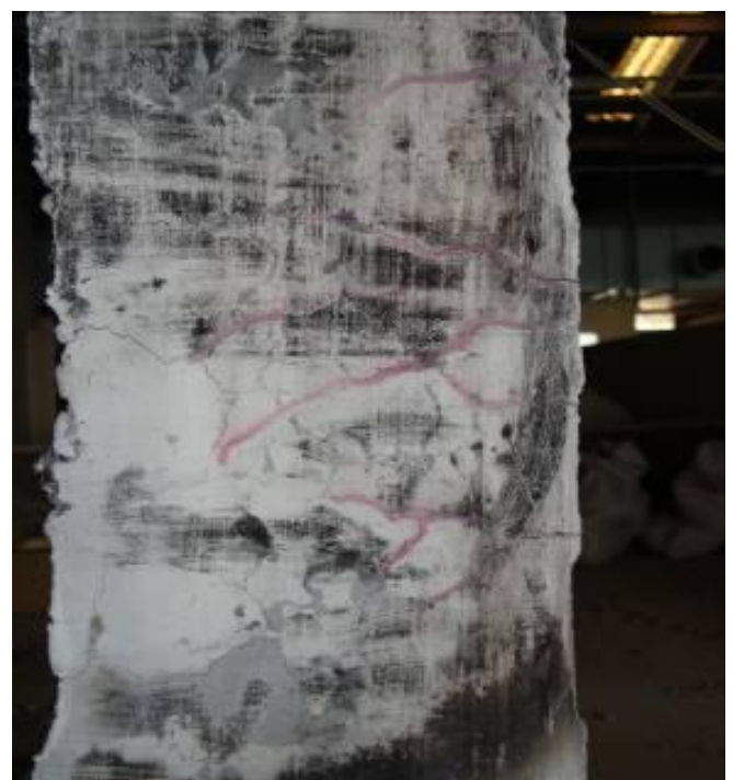
Fig. 16-Formation of transverse cracks due to exposure to fire 1472°F (800°C) and eccentric loading. Note: tC = (tF - 32)/1.8
