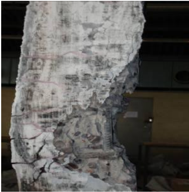
Fig. 17-Formation of triangular-shaped cracks due to exposure to fire 1472°F (800°C) and eccentric loading prior to failure. Note: tC = (tF - 32)/1.8
