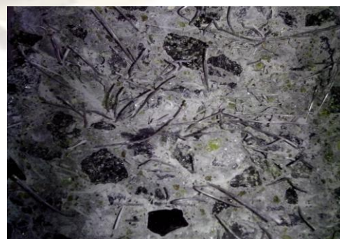
Fig No. 4 Cross section of the beam specimen after ultimate failure.
