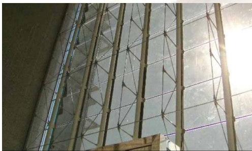
Fig 16: Image of a commercially available "see thru" BIPV Product.
