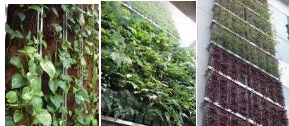
Panel Type Mini planter Cage System Fig 5: Various Green Wall Structures
