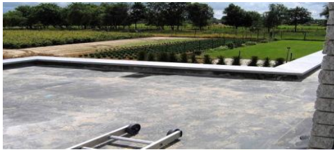
Fig 11: Rubber Roof Structure
