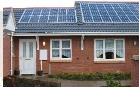
Fig 8: Photovoltaic Roof System
