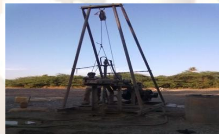
Fig. No.3: Core Drilling
