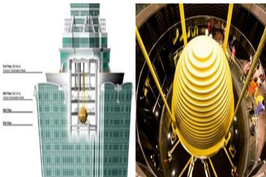
Figure 1. Tuned Mass Damper in Taipei 101.
