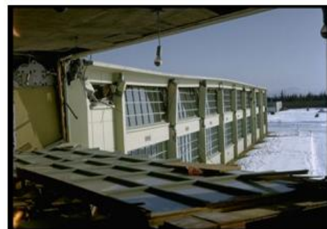
Fig-5 Damage to West Anchorage High School. Window wall fell inwards into the classrooms. Note sag in roof due to failure of reinforced concrete diaphragm during 1964 Earthquake.
