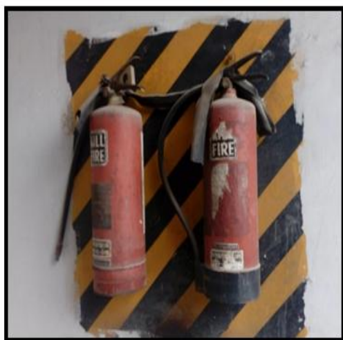
Fig 7 Provision of Fire extinguishers
