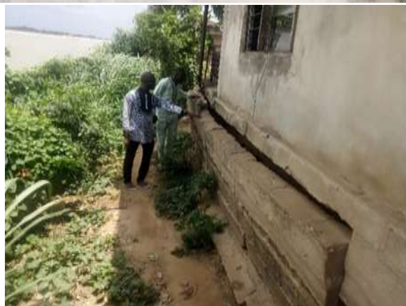
Plate 3: collapsed foundation wall
