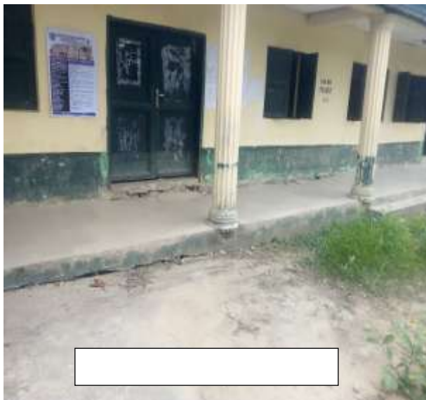
Plate 2: collapsed walls/foundation
