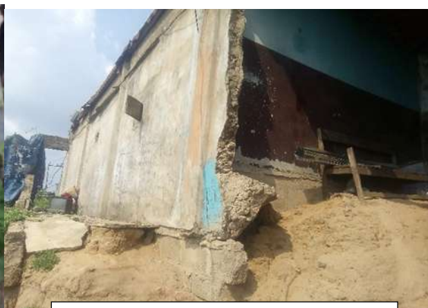
Plate 6: Collapsed wall and foundation
