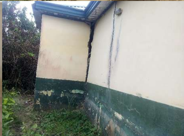
Plate 4: wall separation
