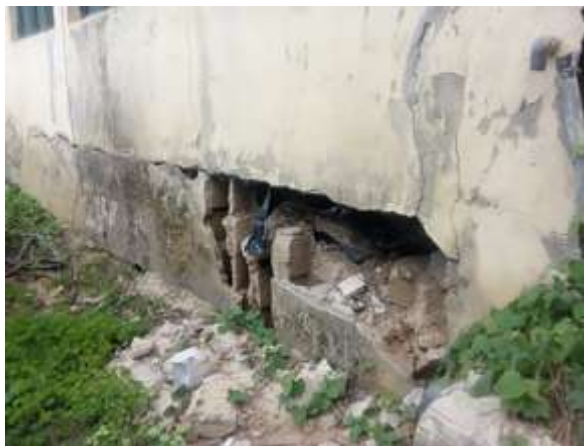
Plate 5: Collapsed foundation wall
