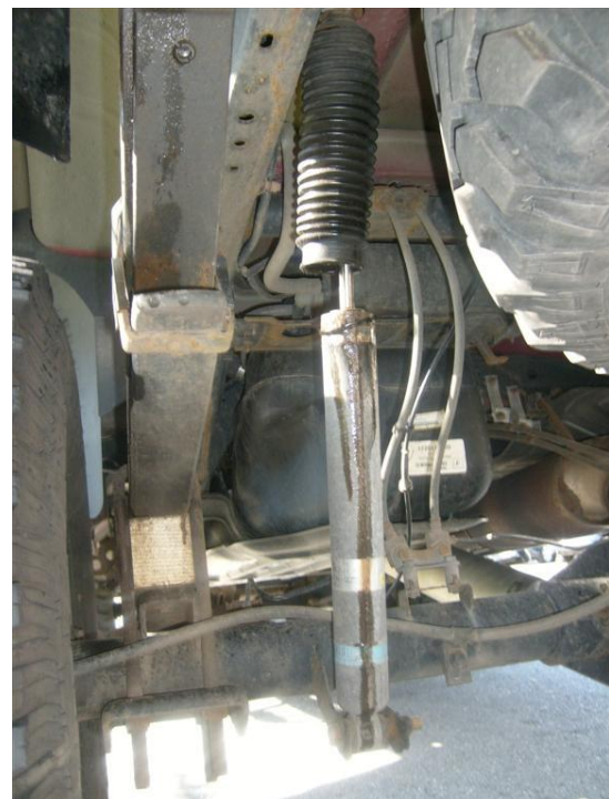
Figure-1: Rear shock leaking (wwundrasolutions.com).
