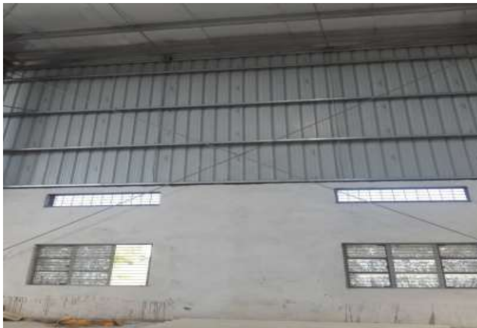
Fig.1 MS rod used as column bracing
