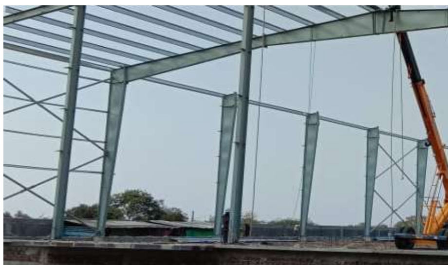
Fig.2 warping of column and rafter web plates during erection
