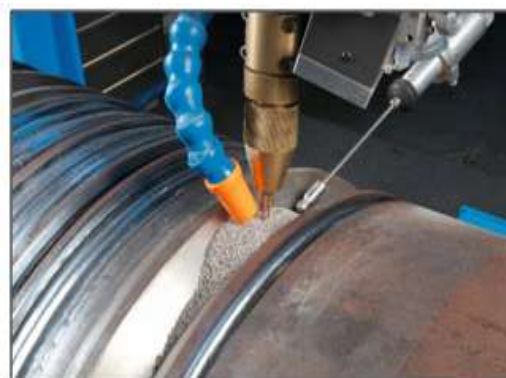
Submerged arc welding
