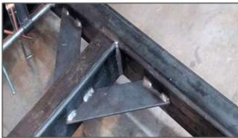
Frame weld joint
