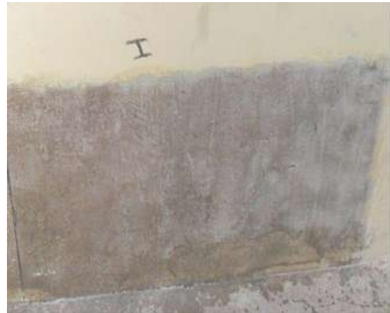
Fig -7: Appearance after sodium silicate coats
