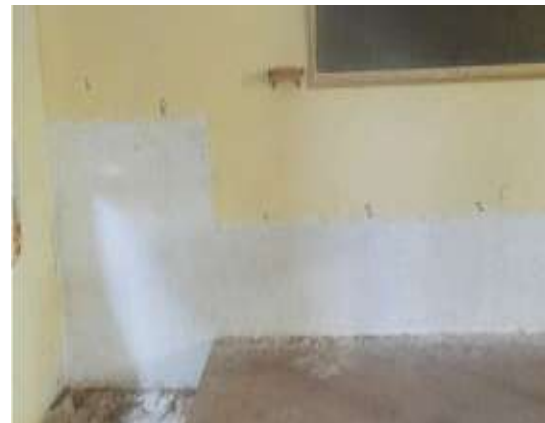
Fig -7: Appearance after white cement coat
