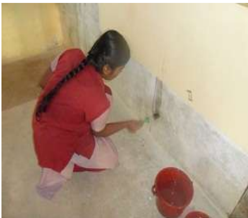
Fig -6: Application of sodium hydroxide solution
