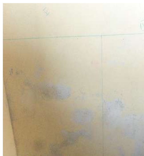
Fig -4: Wall divided into portions
