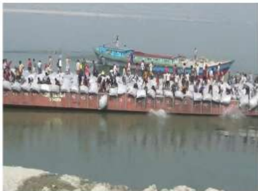
Figure 2.4 : Dumping of geobags
