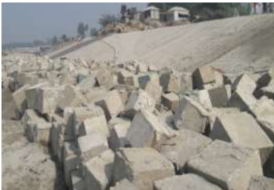
Figure 2.8: CC blocks dumped on loose material
