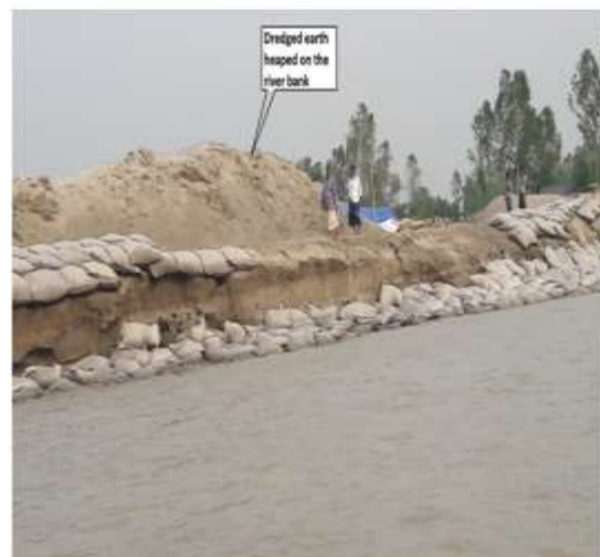
Figure 2.7: Dredged earth heaped on the river bank
