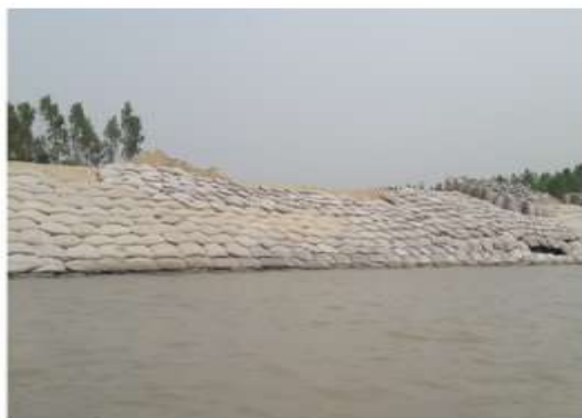
Figure 2.5: Temporary Wave Protection, April 2016
