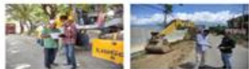
Figure 3 Lagarutu and Main Access road works in Huntap II Housing
