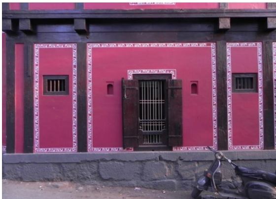
Fig.2. Facade of the temple, timber and brick construction. Image Source: Author
