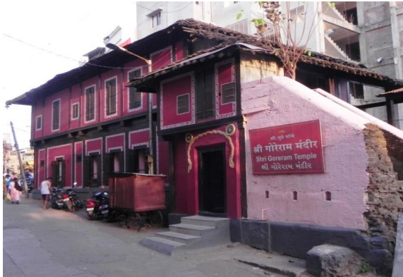
Fig.1- Image showing the exterior and entrance door of Shree Goreram temple, Nashik. Image Source: Author
