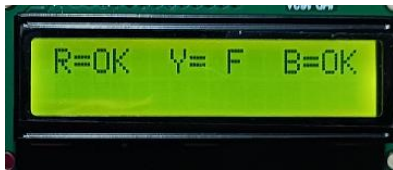
Fig.12: Fault in yellow phase
