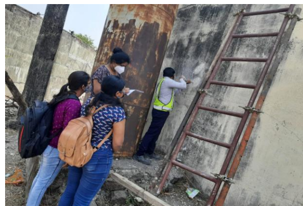
Fig.5 Recording readings of Rebound Hammer Test
