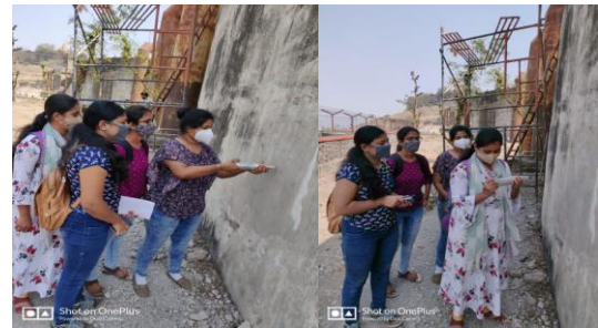
Fig.4 Performing Rebound Hammer Test
