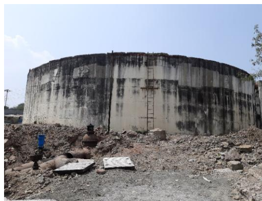
FIG.1 Circular Water tank resting on ground
