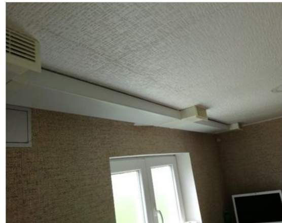
FIG. 13 View of the air ductwork in the measuring room [Photo source: authors]
