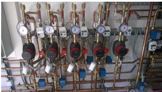
FIG. 11 Distributor and collector with measuring instruments on the heat transfer side [Photo source: authors]
