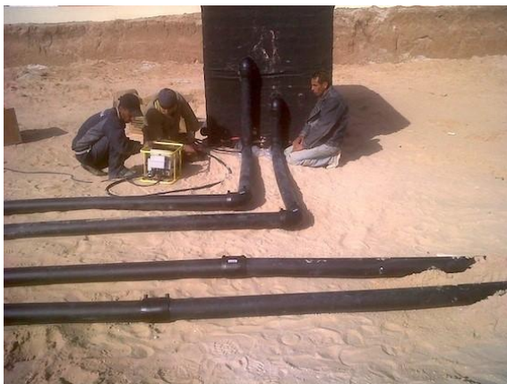
FIG. 3. Construction of the AUM geothermal system.
