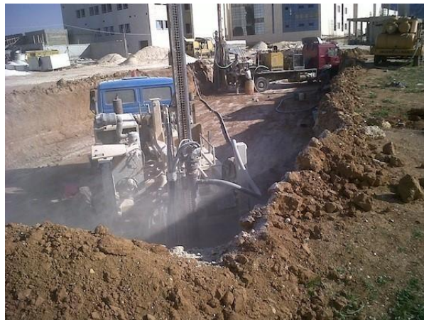
FIG. 4. Construction of the AUM geothermal system (Vertical heat exchanger).
