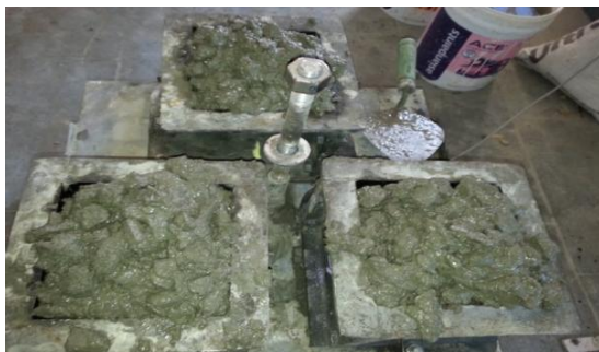
Figure 2: Placing Of Concrete
