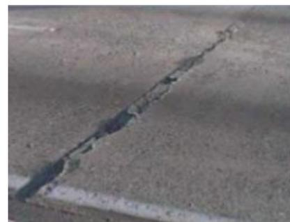
2. Faulting: A difference in elevation across a joint or crack usually associated with undoweled slab. It is noticeable when the average faulting in the pavement section reaches 2.5 mm, when it reaches 4mm diamond grinding or other rehabilitation measures should be considered.
