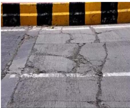
4. Corner Cracking: A crack that intersects the Pcc Slab joint near the corner (within 2m). A corner break extends through the entire slab and is caused by high corner stresses.
