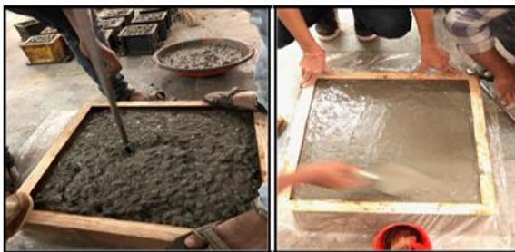
Figure 2. Slabs cast for testing
