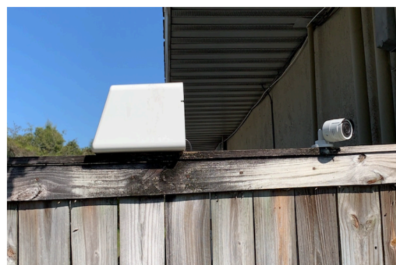
Fig. 5. Installation in Babcock street
