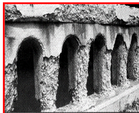
Figure1.2: Freeze Thaw Effect And Cracking In Concrete
