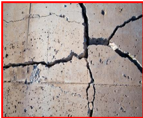
Figure1.2: Freeze Thaw Effect And Cracking In Concrete
