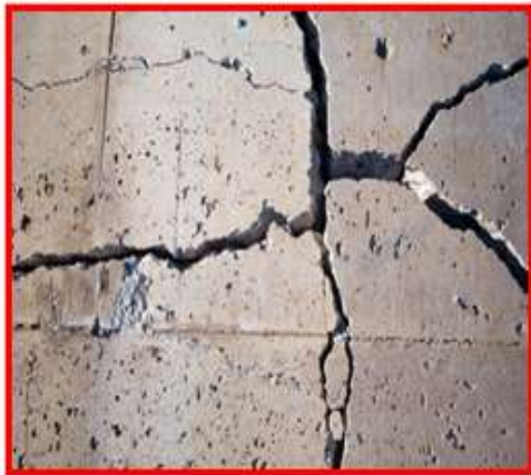
Figure1.2: Freeze Thaw Effect And Cracking In Concrete
