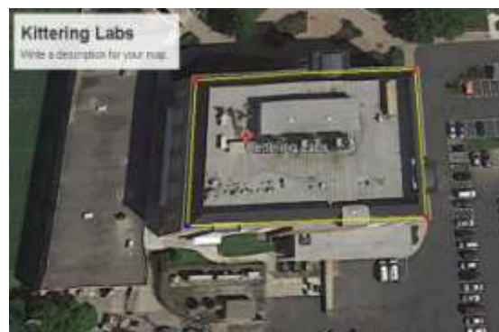
Figure 3: The location of the solar concentrator array system
