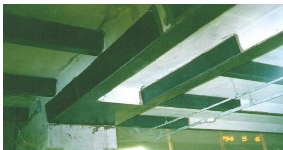
Figure 1. Flexural strengthening of reinforced concrete beams
