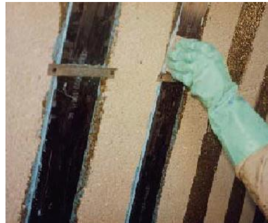
b) application of the laminate
