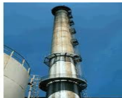
Fig – 1 Cantilever steel chimney
