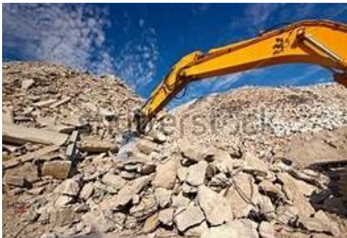
Fig. 1 Construction And Demolition Waste
