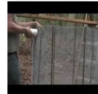
Ferrocement applying mortar
