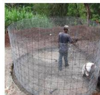
Ferrocement cage fabrication
