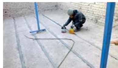
Figure 4. Galvanized protection on the Dârüşşifâ after sanding [5]
