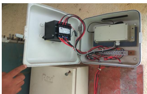
(a) FFig4. Energy Meter for actual time monitoring of grid
