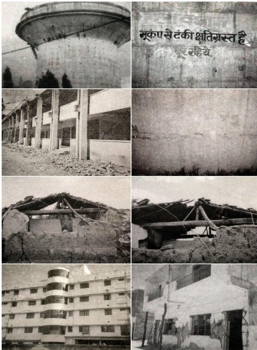
Figure 6 Pictures of some structures built on reclaimed lands damaged in 1997 earthquake in Jabalpur M.P.
