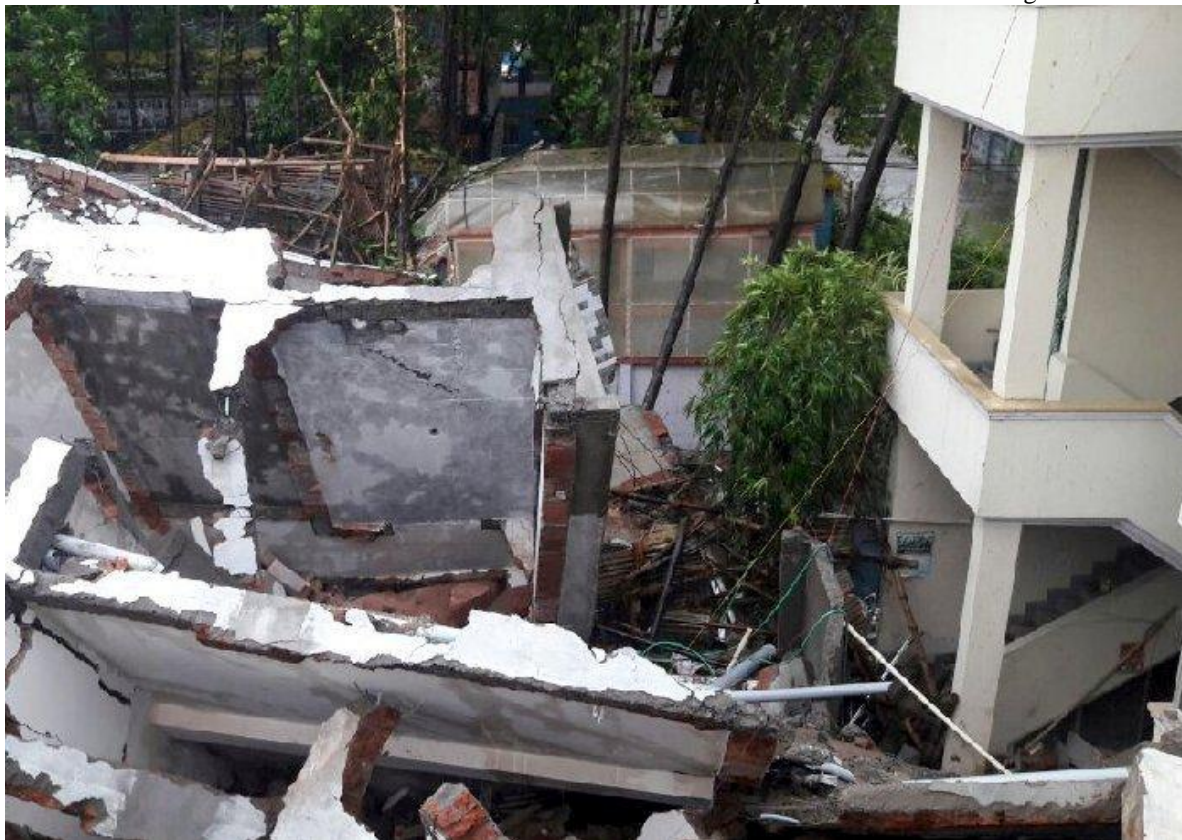
Figure 5 A seven storey building collapsed near Cherital Lake in Jabalpur
