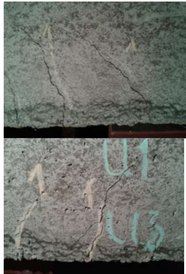
Fig.3 The next crack on front and both sides
