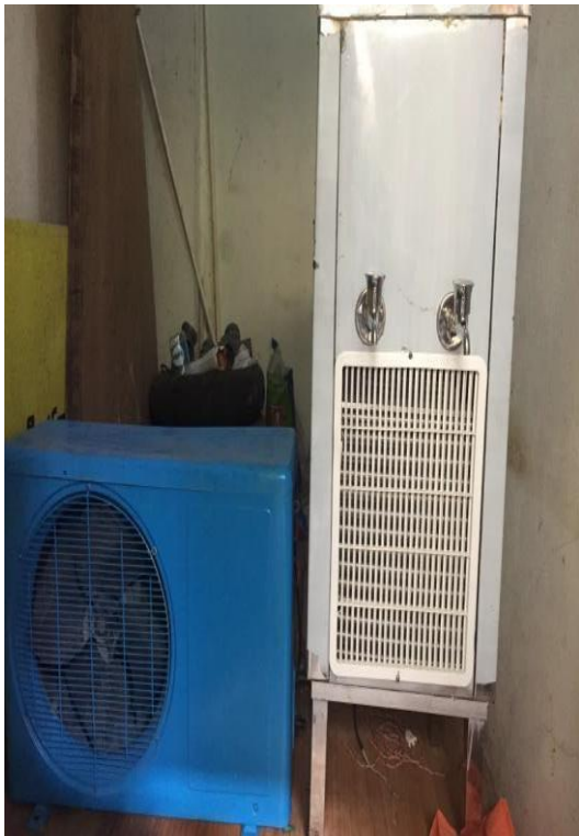
Water cooler cum air conditioner
