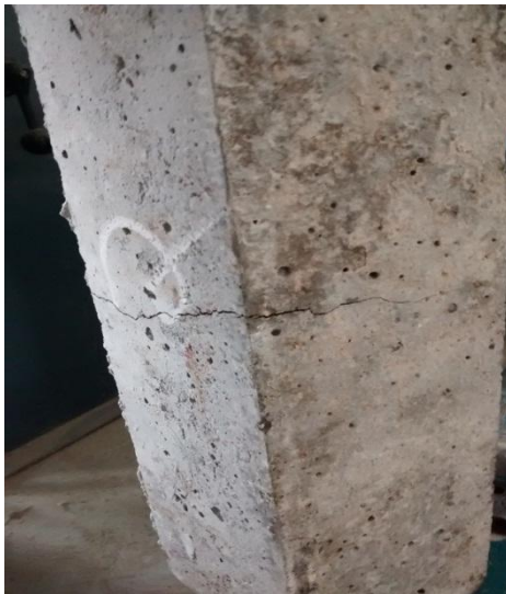
Fig 8 Beams showing crack before failure
