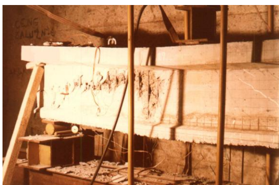
Fig.3 The cracking of the beam
