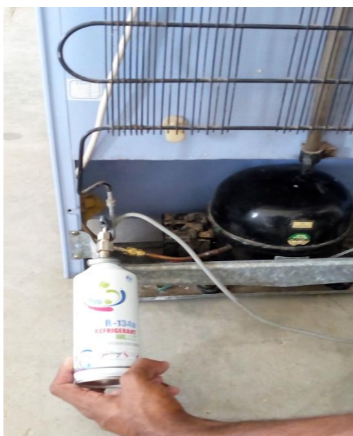
Figure 3 refrigerant charging vessel
