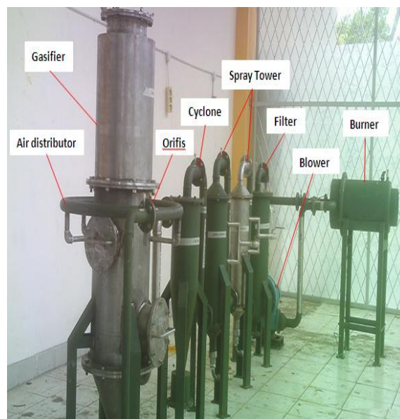
Figure 8. The Construction of Gasification System
