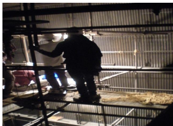
Fig. 4 - Scanning of water wall tubes
